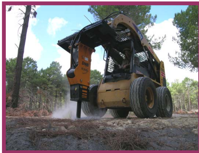
Don Sherlock testing the Rock Breaker
